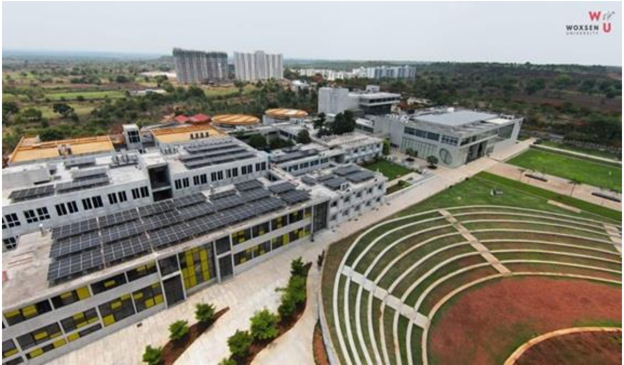
420 kWp Solar Setup (Phase -2)
